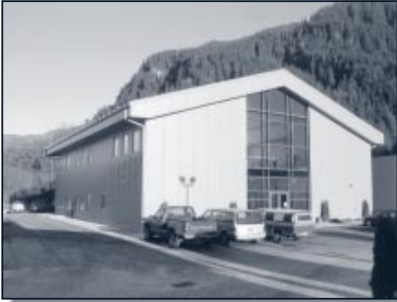
Southeast Alaska Tribal College Campus, Juneau
